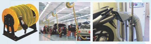
Vehicle exhaust / Engine extraction systems normally involve the collection and extraction of exhaust gases at significantly higher temperatures than those generated from standard passenger cars. This increase in exhaust gas temperature is due both to the greater power outputs of the engines under test and the fact that in the majority of cases, engines are run on rolling road or fixed dynomometer under full load.
